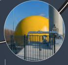
There are special bacteria in the bioreactor which multiply and eat waste, which then decomposes to produce biogas. The separated biogas is collected and used to generate electrical and heat energy, which are needed for the remaining processes.
